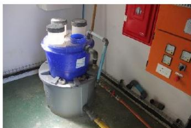
Klorman Disinfection currently used
