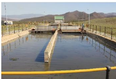
Pasveer Oxidation Ditch
