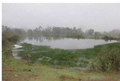
Primary Aerobic Pond No. 1
