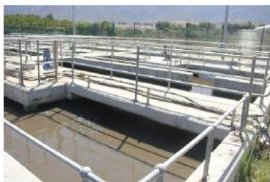
Reactor: Anaerobic Zone
