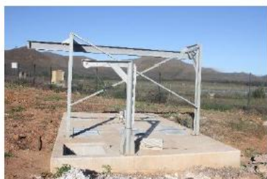
Raw wastewater PS
