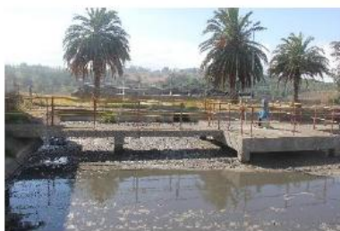
Reactor: Anaerobic zone
