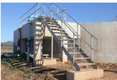
Raised Inlet structure
